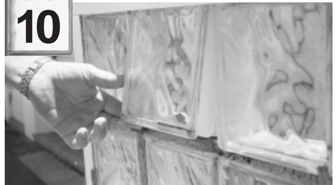
The last touch. Insert Glass Blocks at each end working towards the centre. Joint with roller jointer. Sponge off with wet sponge. Leave to dry until a white film appears on the glass blocks. Final jointing can then be done. White film can be cleaned off with a dry sponge or duster.
