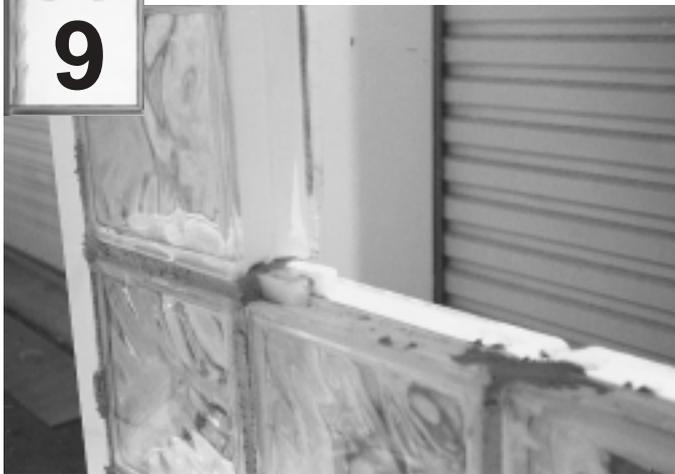
When placing the last row of glass blocks use jamb connectors only, inserting flat side up.
