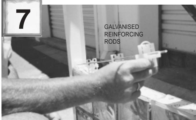
Cut galvanised reinforcing rods to length and thread through holes in connectors. Push into place between blocks. Two reinforcing rods to be used in every two horizontal row of blocks throughout wall height.
