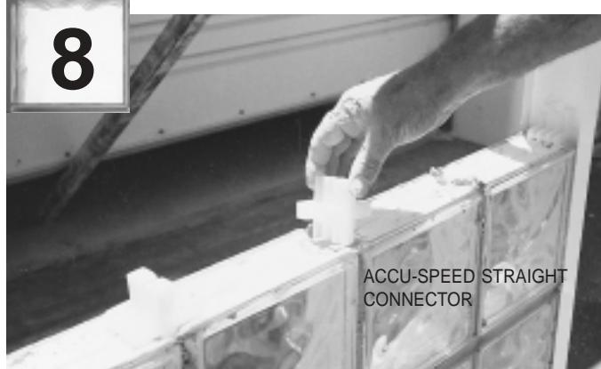
Place mortar between connectors and repeat laying procedure, remember keep mortar flush with connector to ensure glass block sits tight.
