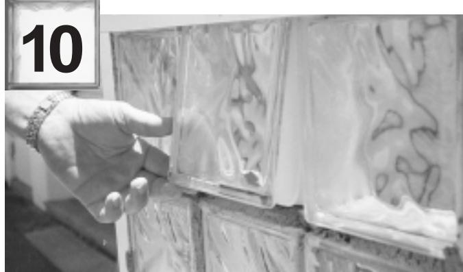
The last touch. Insert Glass Blocks at each end working towards the centre. Joint with roller jointer. Sponge off with wet sponge. Leave to dry until a white film appears on the glass blocks. Final jointing can then be done. White film can be cleaned off with a dry sponge or duster.
