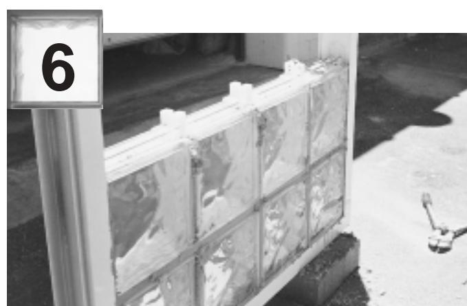
Repeat for second course using straight connectors with jamb connectors at each end.
